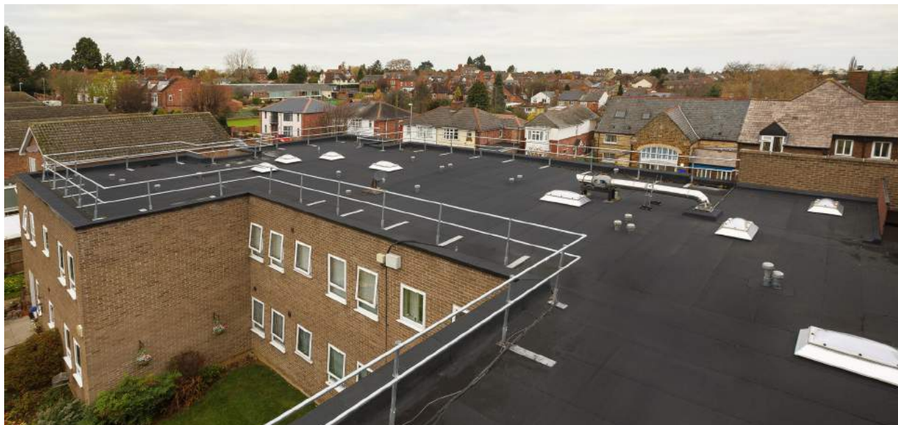
Hatton Hall Sheltered Housing, Wellingborough, Northamptonshire Size 750m 2 The project was to refurbish the roof, improve drainage and insulation and bring it up to current building control standards. IKO UPXL was primarily chosen by the client for the 30 year single-point guarantee. Contractor: Breyer Group PLC System: Reinforced Bituminous
