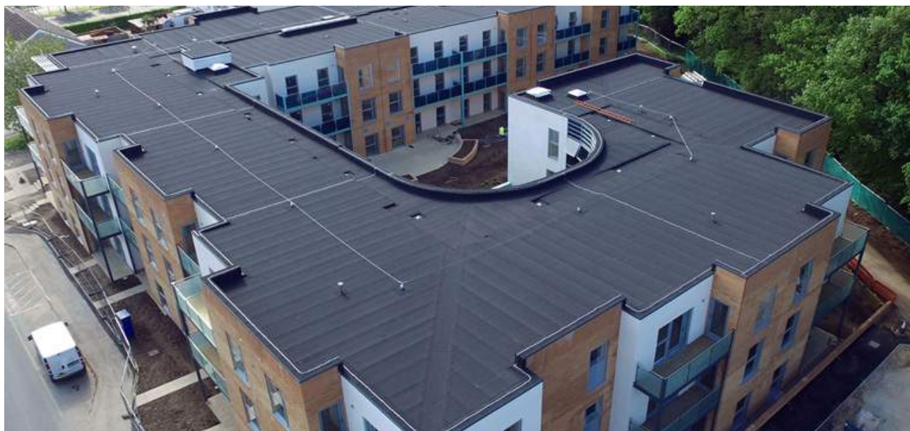
Erskine Court, Southampton Size 2,000m 2 A waterproof roofing system was required that would provide a long-term solution and deliver quality and value for money for a new housing development. IKO UPXL system offered a 30 year single-point guarantee which was paramount to the project. Contractor: Salnor Roofing Services Ltd System: Reinforced Bituminous
