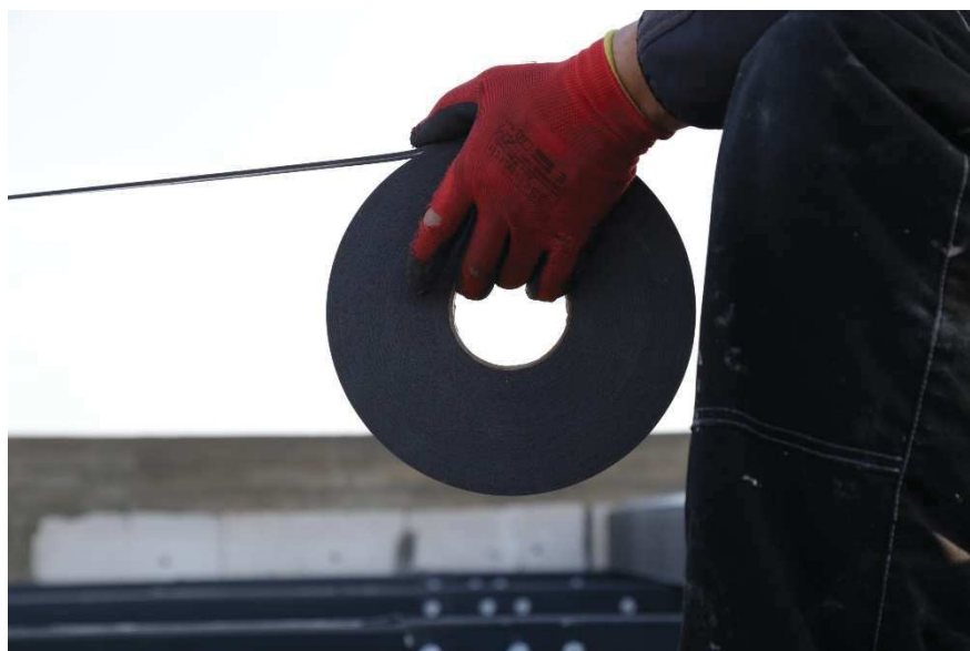
2) APPLICATION OF THE PES SEALING TAPE TO THE SUBSTRUCTURE SUPPORT ELEMENTS
