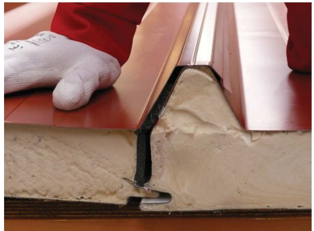
Right: the process of pressing in the joint lock profiles between PU-R 40 sandwich panels (not applicable to sandwich panels with double tongues)
